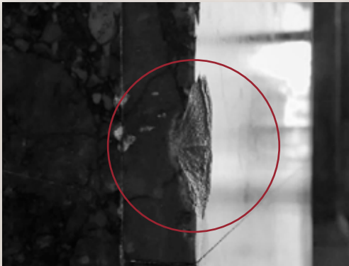
BULLET HOLE: The only remaining evidence of a gun battle which took place at Central Station in 1916 is a small bullet hole in the marble (circled) by the entrance to Platform 1.
