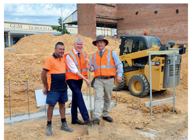
SOD TURNING: With Grenfell medical centre site foreman John Anderson (left) and Weddin Mayor Mark Liebich.
