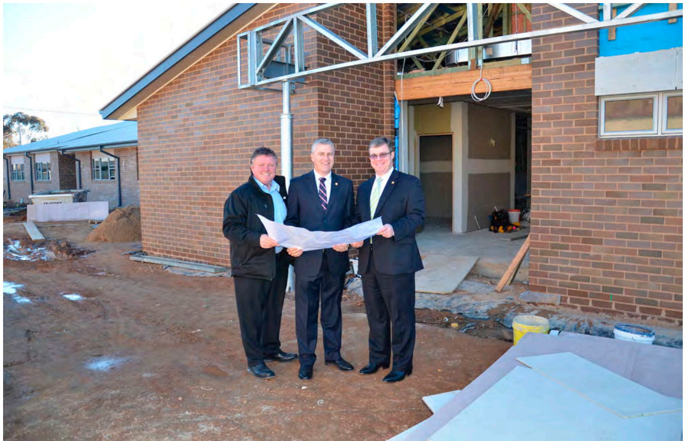
BIG PLANS: Looking at the building blueprint for the new Temora Medical Complex with Temora Shire Council General Manager Gary Lavelle (left) and Chairman of the Council's Health Strategies Committee Cr Rick Firman, who is also Temora Deputy Mayor.
