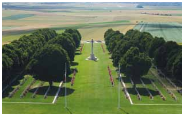
NOW AT PEACE: aerial photograph of Villers-Bretonneux just east of Amiens, France, where Wyalong's Stephen Lonergan, having fallen in The Great War, is memorialised.
