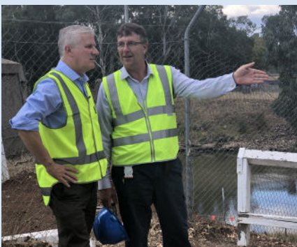
PROTECTING WAGGA WAGGA: Inspecting levee bank upgrade work in March with Wagga Wagga City Council Senior Project Manager Darryl Woods.
